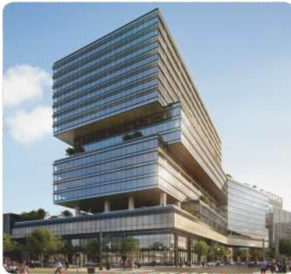
Reference Image of Gateway Building
